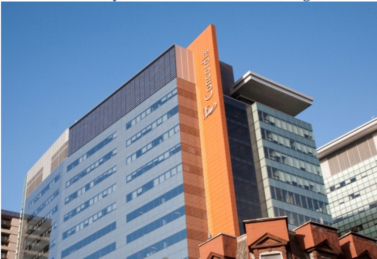
Fig 1. (a) Street view of JMSB solar system
